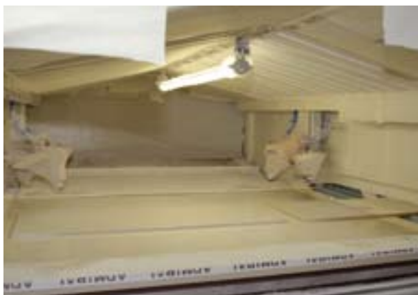
The modern paint-spray line, fully automated.
