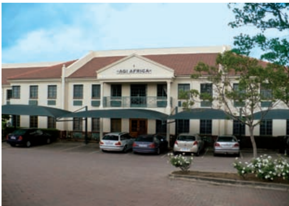
AGI Africa headquarters in Midrand, Gauteng.
