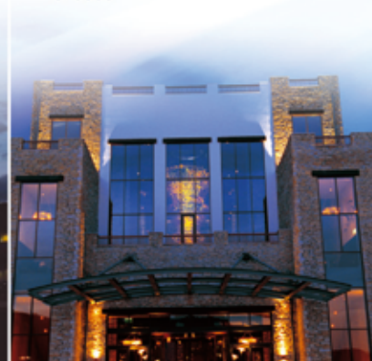
Regency Casino Mont Parnes, Greece
