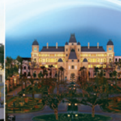
GrandWest Casino, South Africa
