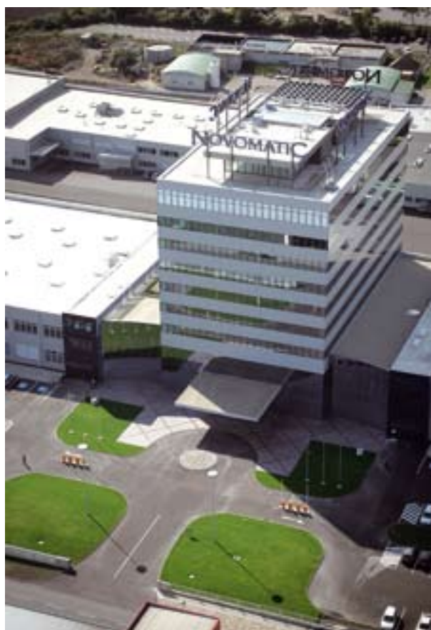
Novomatic Headquarters in Gumpoldskirchen.
