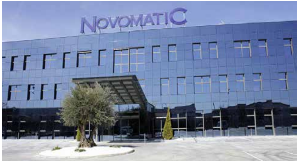
NOVOMATIC Spain headquarters in Madrid.
